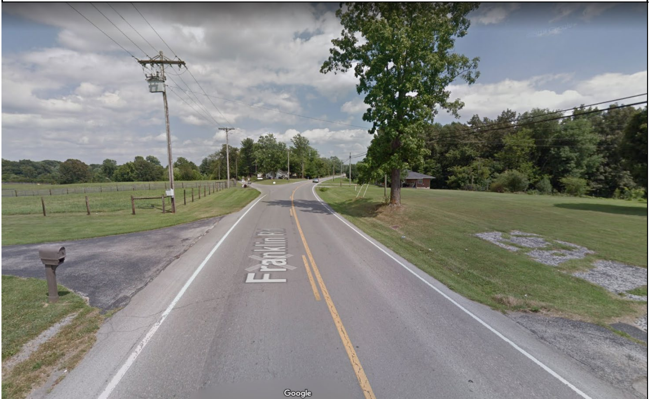
Photo 1: Beginning of the project near the Oliver Street intersection facing east toward Scottsville
