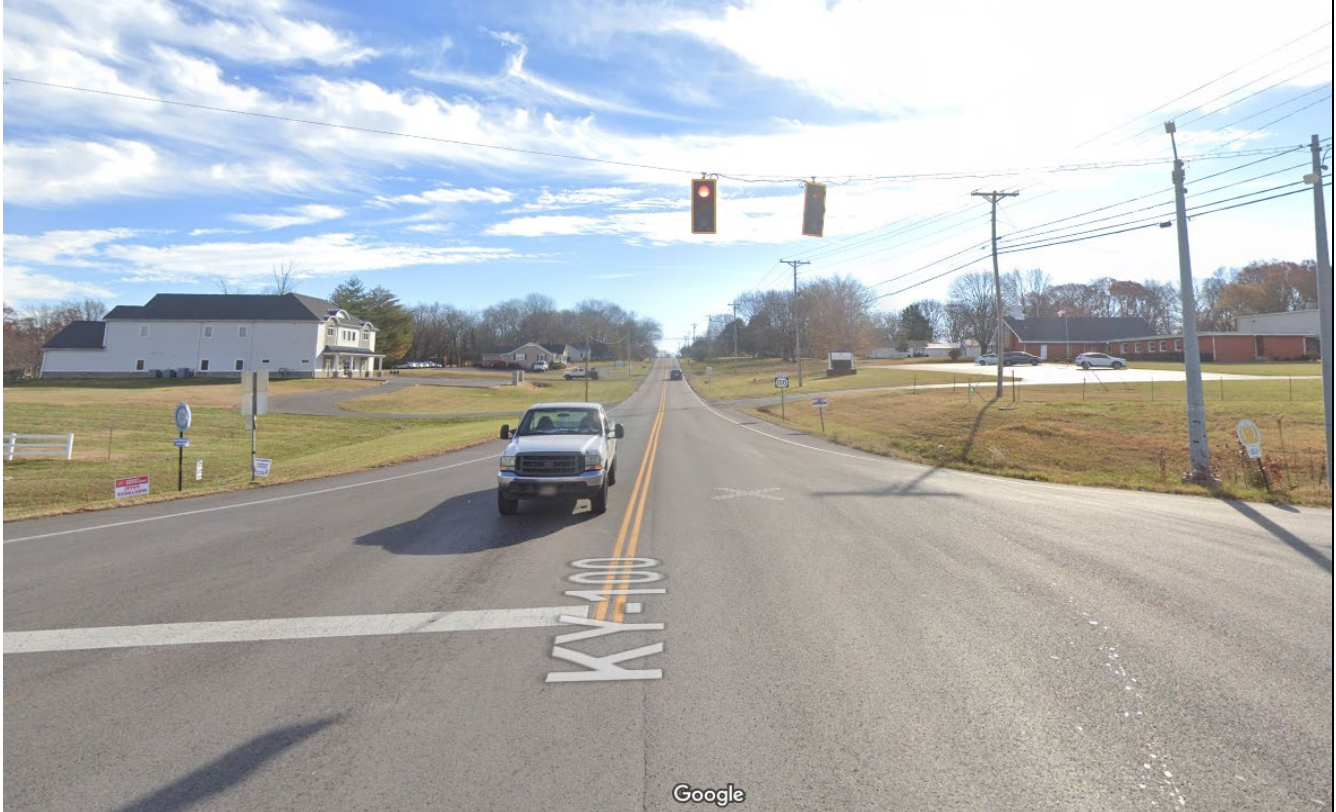
Photo 2: End of the project at the US-31E intersection facing west toward Franklin
